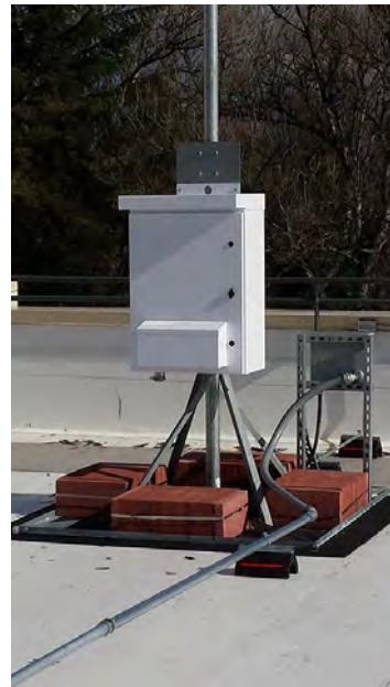
Ground station site construction NEMA enclosure, non-penetrating roof mount w/ ballast
