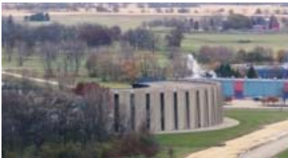
View of Feynman Data Center from Wilson Hall's 15 th Floor.
